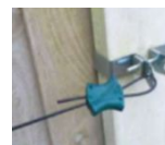
Wire Anchor fitted with Gripple System
